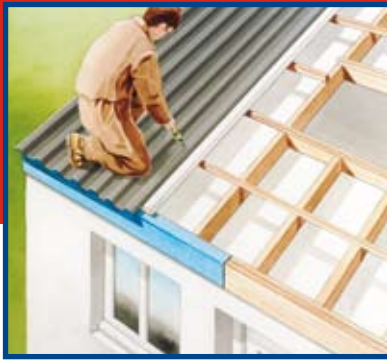
DURING - NEW ROOF BEING FITTED WITH INSULATION
