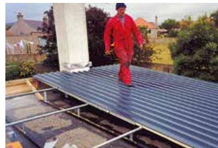
PERMAROOF - strong enough to be walked on
