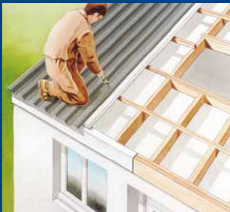
DURING - NEW ROOF BEING FITTED WITH INSULATION
